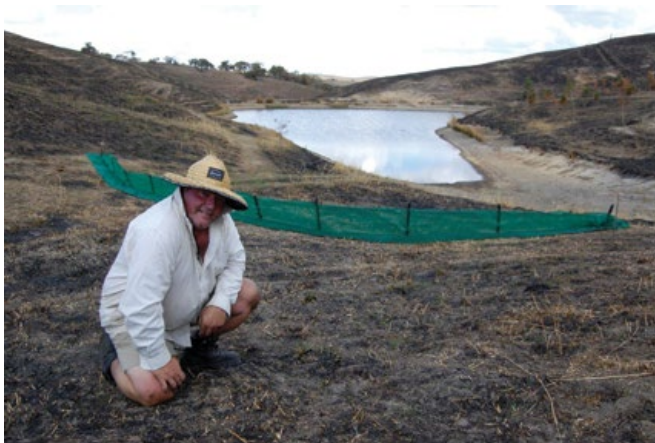
Figure 5.1: Sediment fence built to protect dam from debris and pollution after fire.
